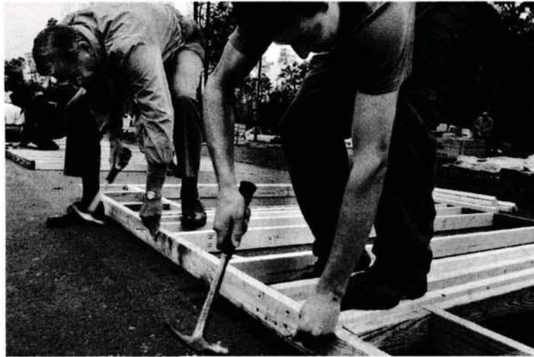
Habitat for Humanity volunteers build a house for people in need.
