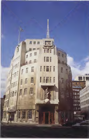
Broadcasting House, headquarters of the BBC
